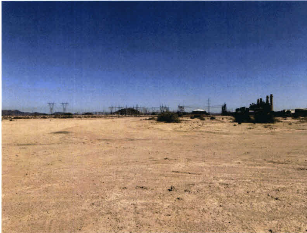
View of existing Redhawk Power Plant and Switchyard looking north from southern boundary near railroad.
